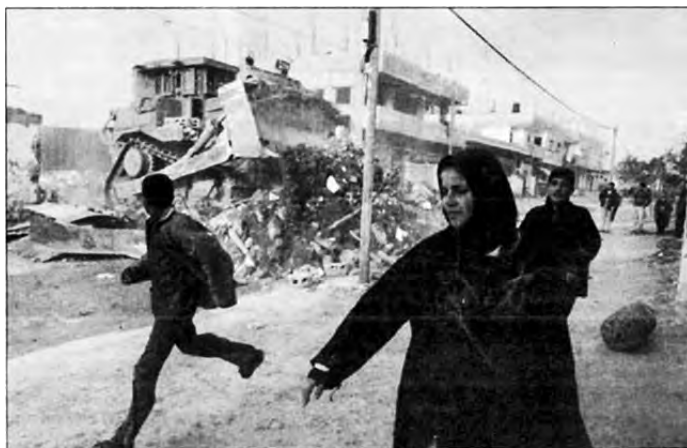
• Military bulldozers in use to bulldoze Palestinian homes
